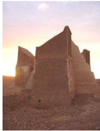
Figure 30 – Photograph of cistern
